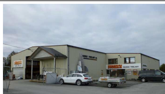
Figur 10: Fauske Trelast AS (Bygger'n).
